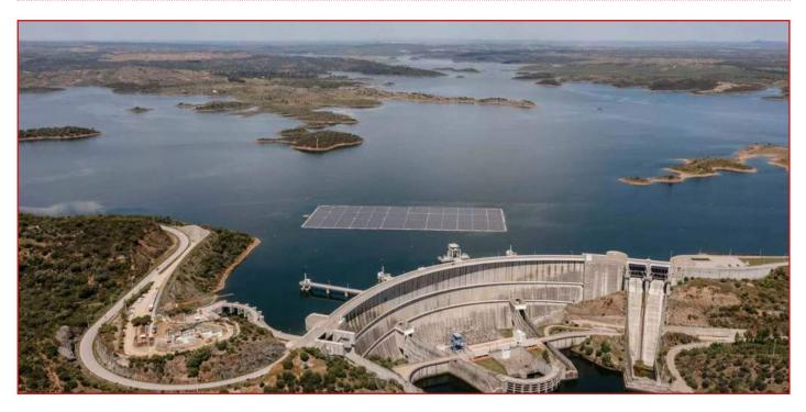
Floating solar farms are a new and effective development in eco-friendly technology that utilise lakes and oceans to host solar panels. They produce up to 20% more energy compared to normal solar panels on land as they are able to track the sun throughout the day, allowing them to catch more sunlight.
